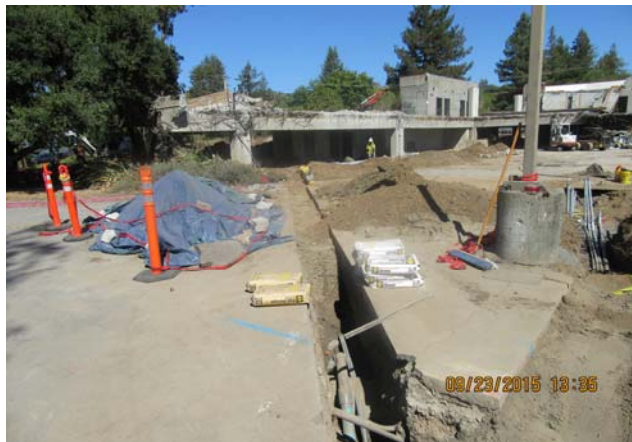
Demolition and underground utility work
