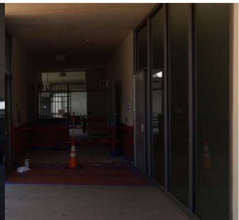
Slip resistant surface application at entry adjacent to courtyard
