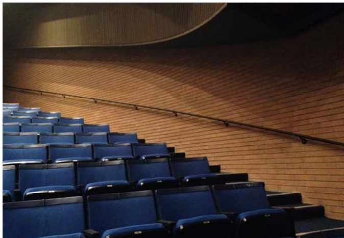
New interior handrails in James Dunn Theatre
