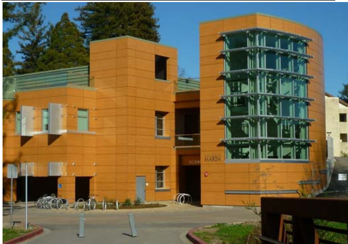
West stair tower and entrance
