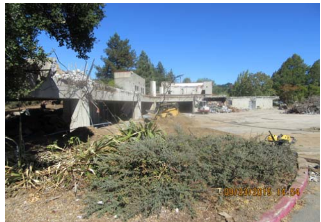
Demolition looking north
