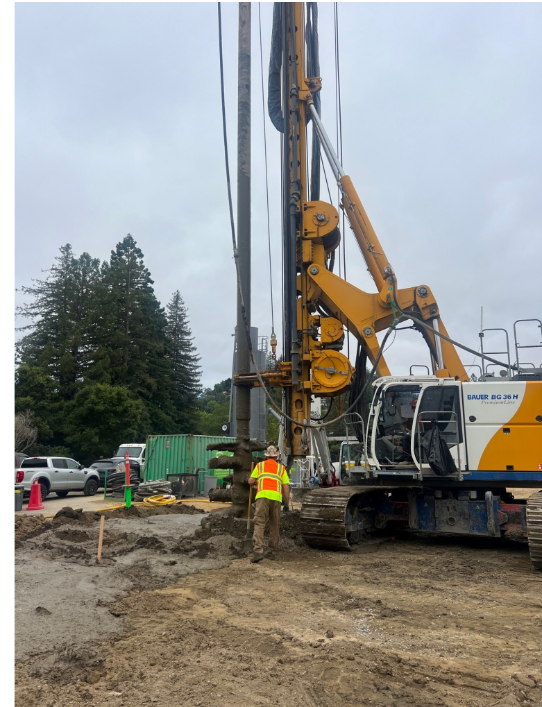
CDSM auger on LRC site
