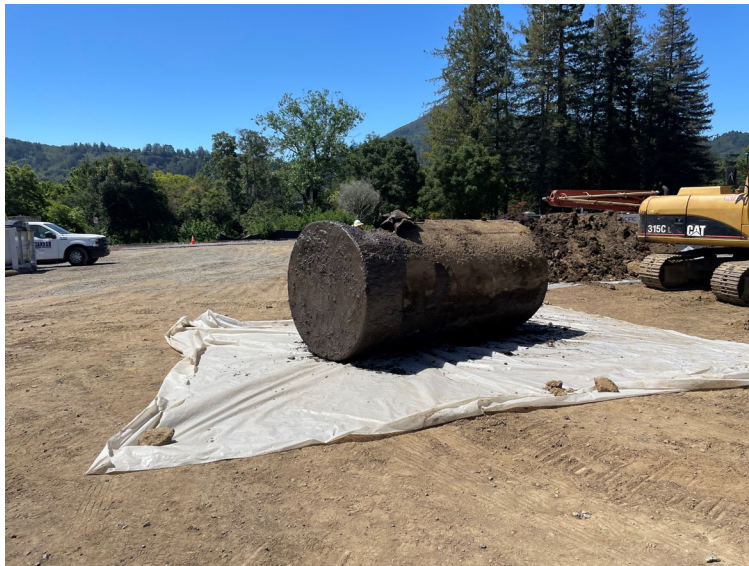
Large Underground Storage Tank
