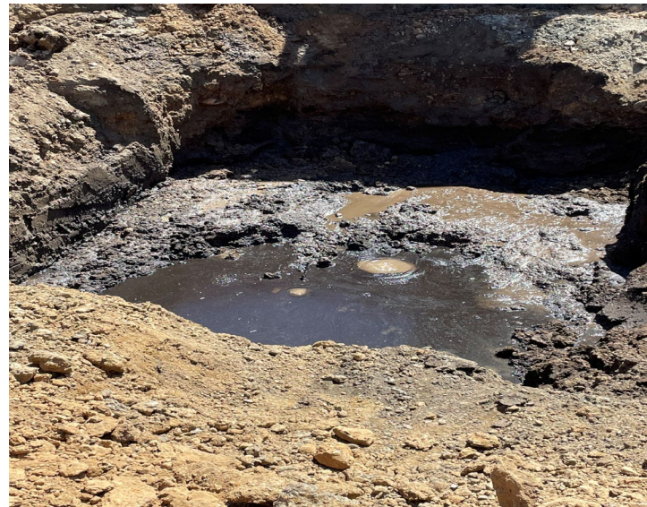
Liquefaction of site - Hole from tank filled with water from Bay
