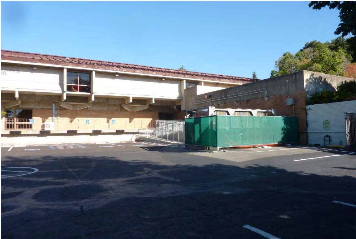
8. East Elevation at Mechanical Room
