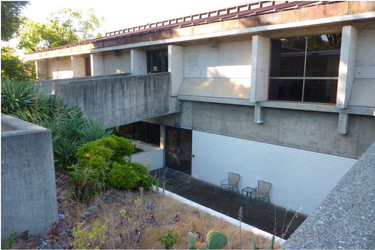
5. North Elevation at East End
