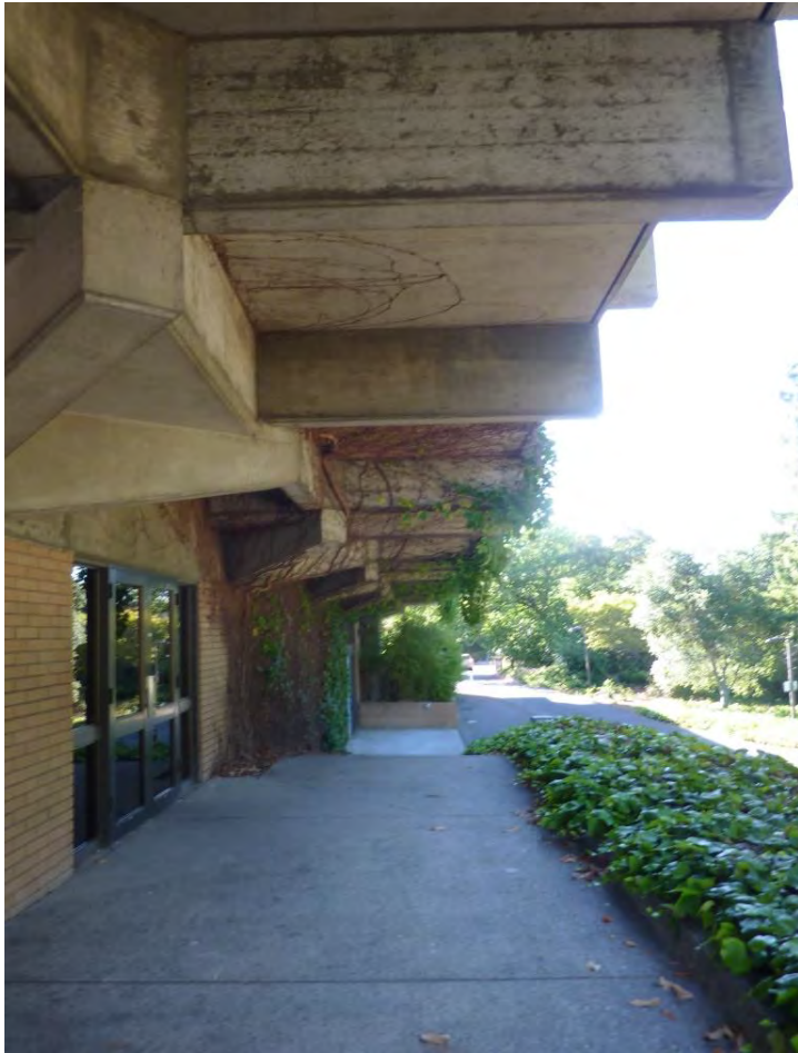
12. South Side looking East
