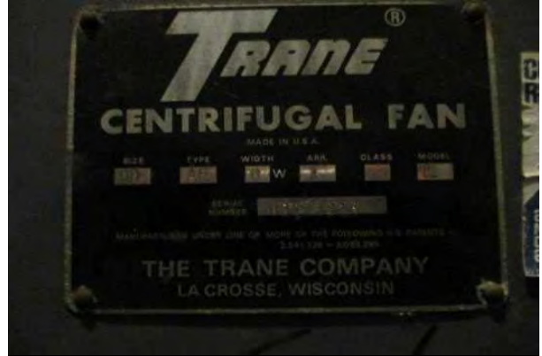
#32: AIR HANDLER, INTERIOR
