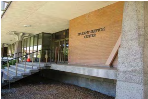
#10: EXTERIOR WALL, BRICK VENEER
