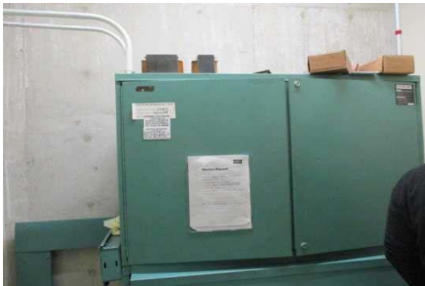
#21: ELEVATOR EQUIPMENT, HYDRAULIC
