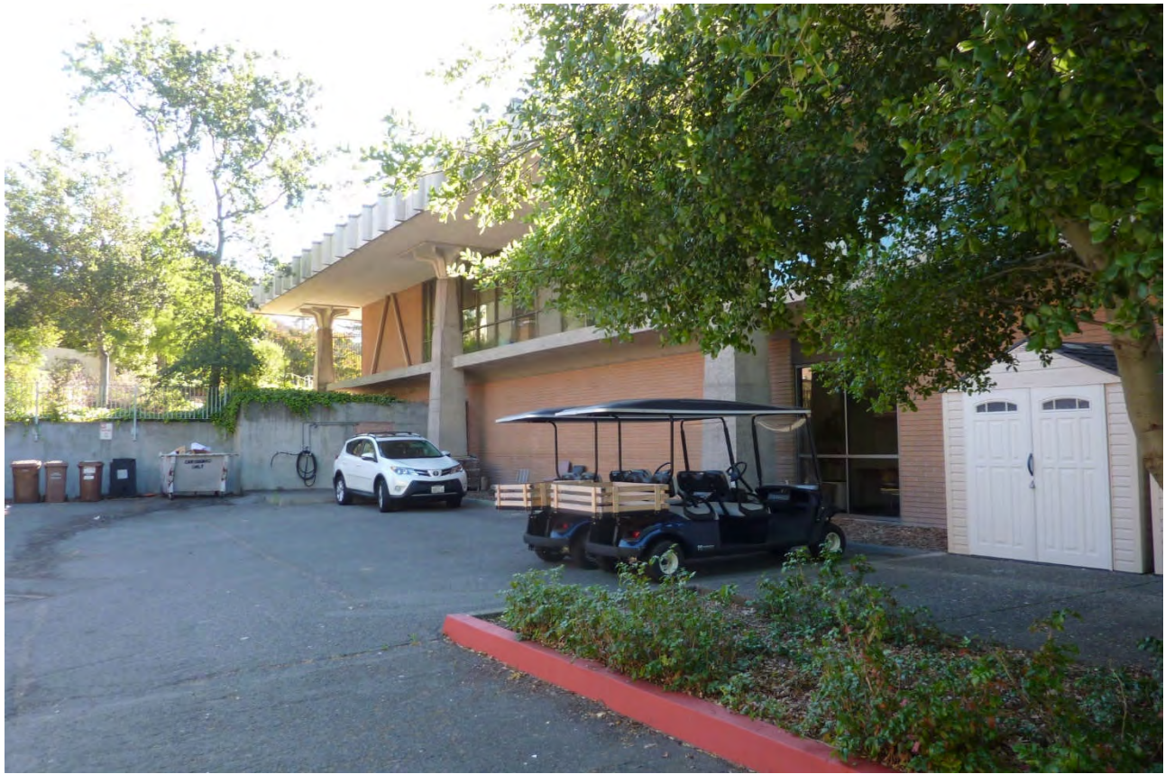
4. West Elevation looking North
