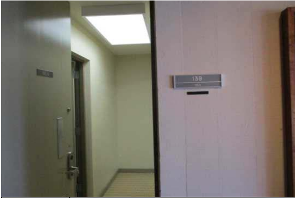
#19: INTERIOR WALL FINISH, PAINT
