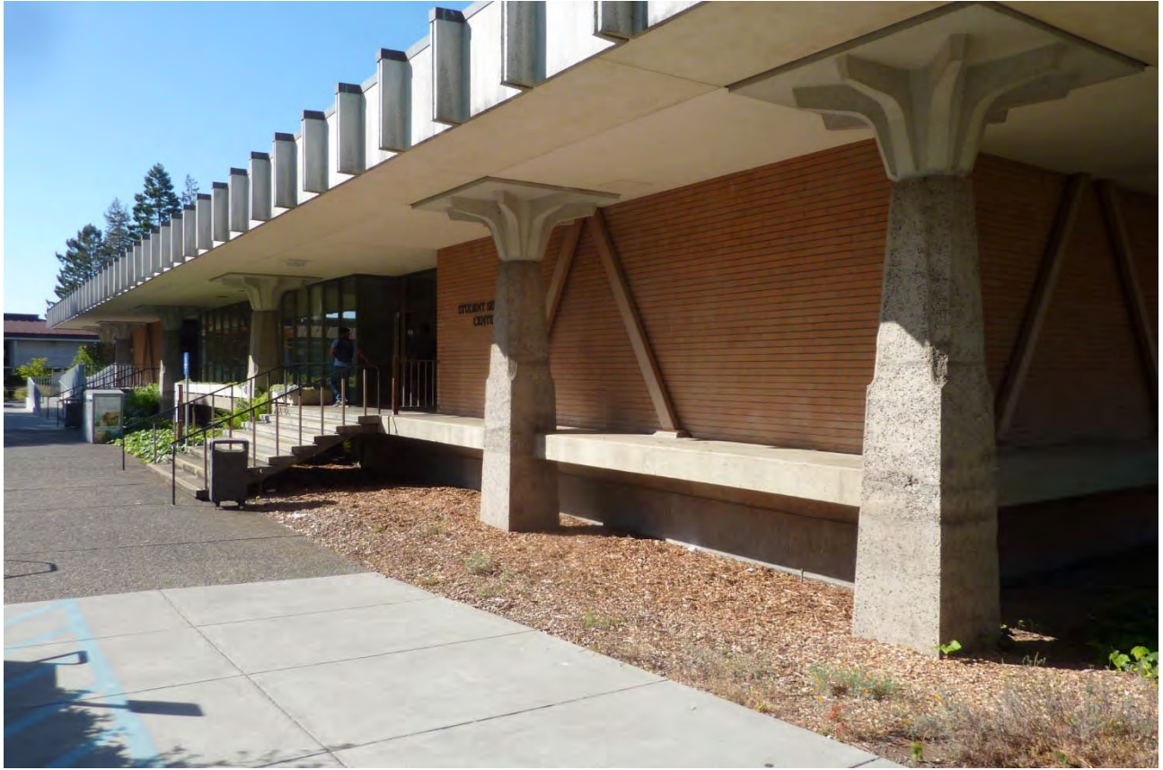
6. Steel Bracing at Northwest Corner
