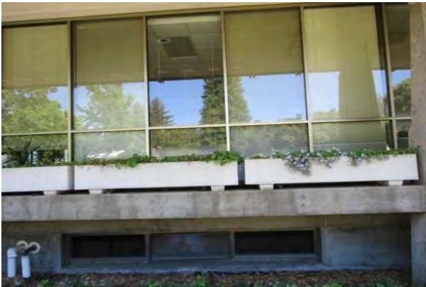
#9: EXISTING SINGLE GLAZED WINDOWS
