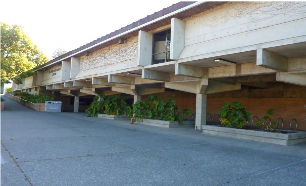
13. West Elevation looking North
