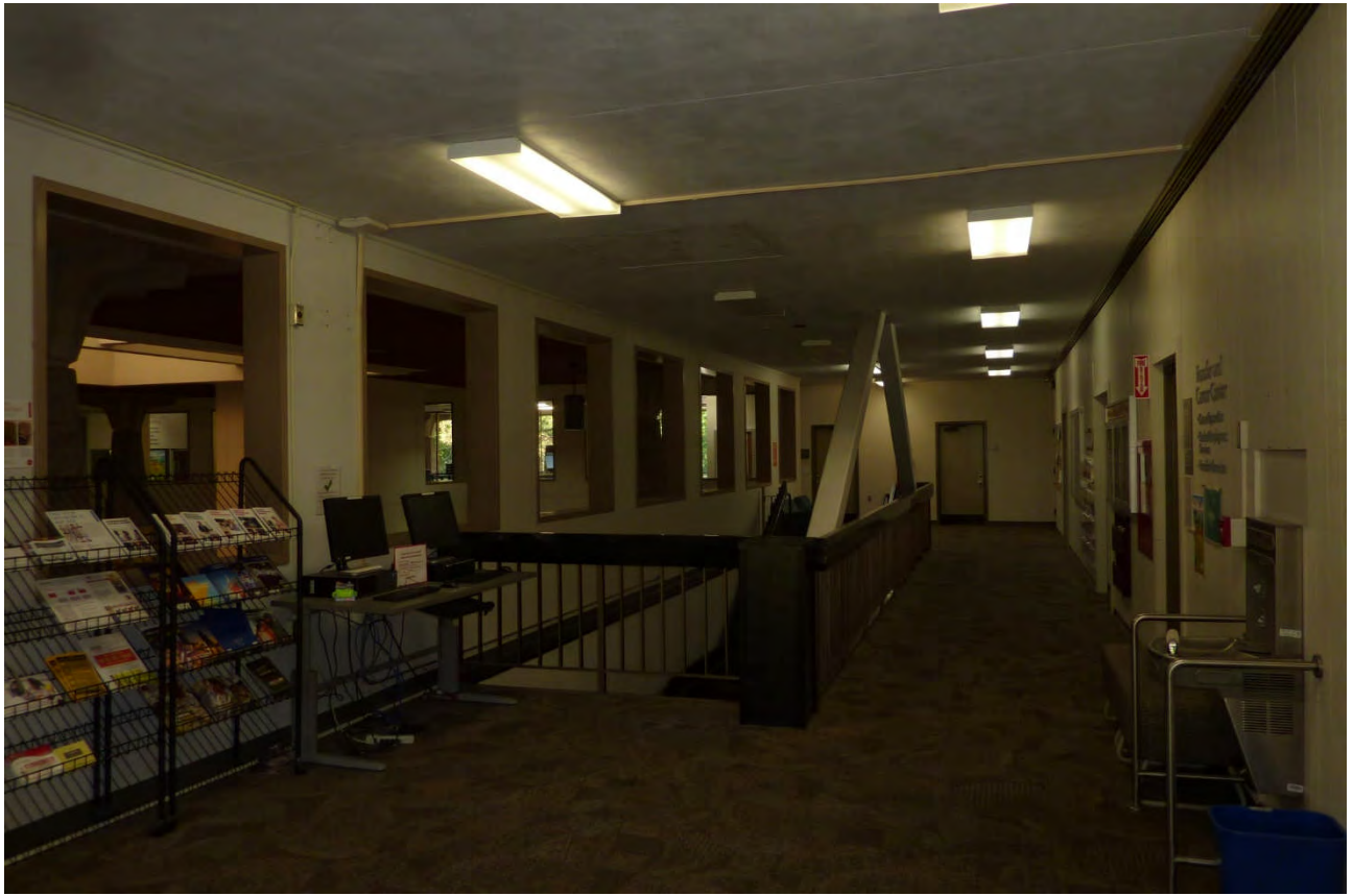
8. Steel Bracing at West Side of Atrium
