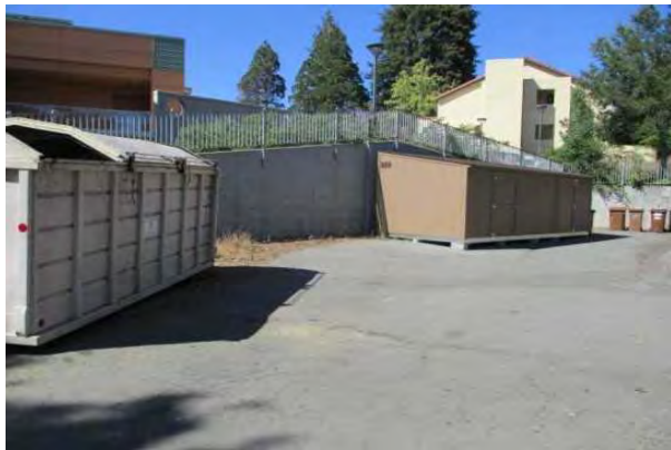
#48: ROADWAYS, ASPHALT PAVEMENT
