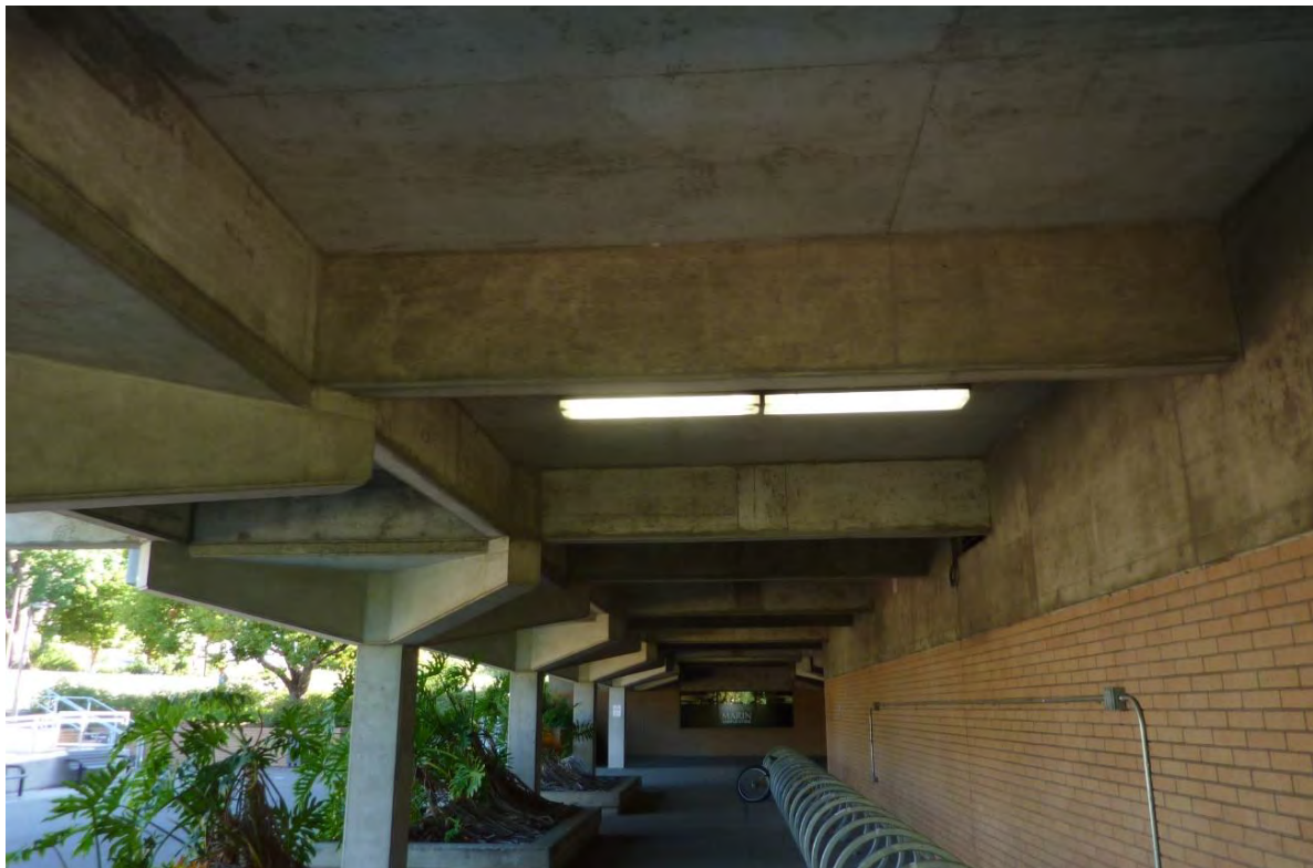
11. Corridor along East Side looking North
