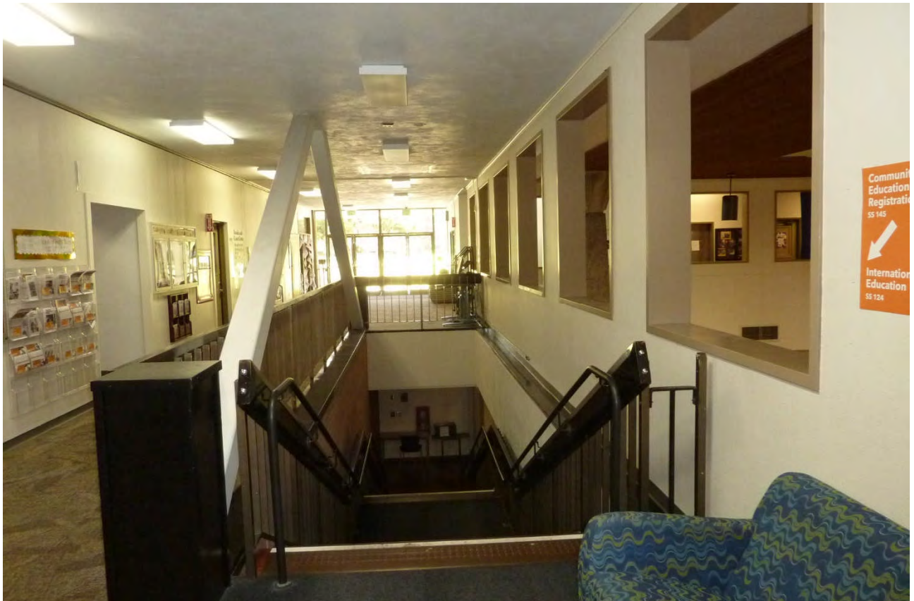
9. Steel Bracing at East Side of Atrium
