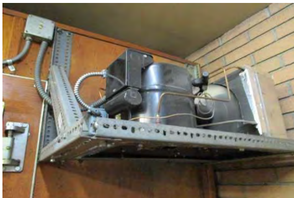
#24: INTERIOR FINISHES, WALK-IN REFRIGERATOR
