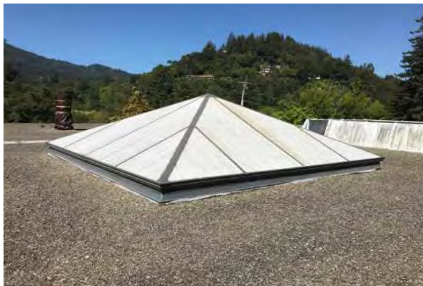
#12: ROOF SKYLIGHT, GLASS SINGLE UNIT
